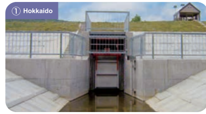
① Hokkaido Oketo Sluice No. 11 (1.20 m × 1.30 m) Orderer: Abashiri Development and Construction Department, Hokkaido Regional Development Bureau
