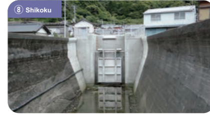
⑧ Shikoku Sluice No. 55 (2.00 m × 2.00 m) Orderer: Susaki City, Kochi Prefecture
