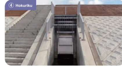
④ Hokuriku Motonakago Sluice (1.20 m × 1.30 m) Orderer: Shinanogawa River Office, Hokuriku Regional Development Bureau
