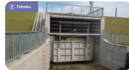
Kotsunagi River Drainage Sluice (4.70 m × 2.30 m) Orderer: Noshiro River and National Highway Office, Tohoku Regional Development Bureau
